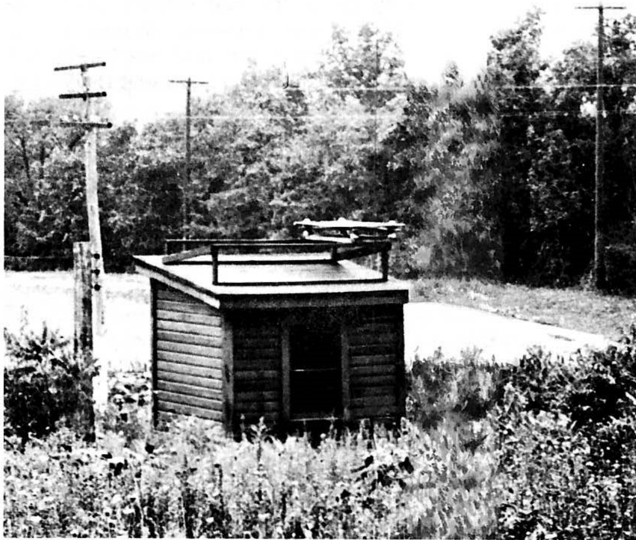
FIG. 1-5. View of air capacitor for field-intensity recorder, mounted on top of wooden house in which recorder is located.
