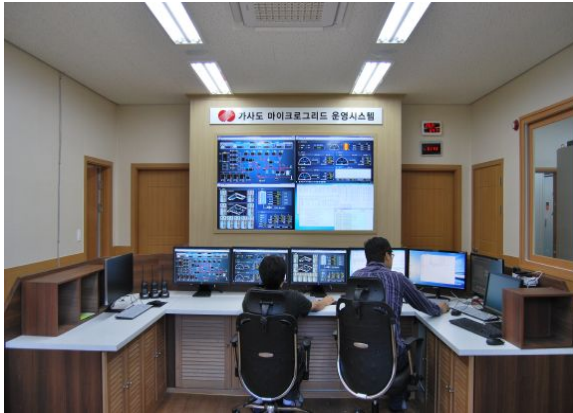
<Gasa-island Remote MicroGrid (Energy Management System , Wind/Solar farm, operation HMI* from left)>
