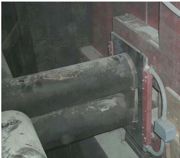
Figure 11. Split-Core Style PCB Rogowski Coils (installed around water-cooled secondary conductors of an EAF transformer)
