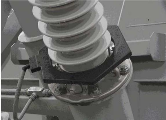
Figure 9. Bushing Type Multi-layer PCB Rogowski Coil Design (installed around bushings of a mobile substation power transformer)
