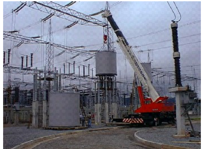
Figure 4 - FURNAS 362kV CLR at site during erection.
