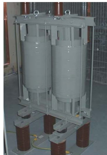
Fig. 1. Filter reactor with two coils
