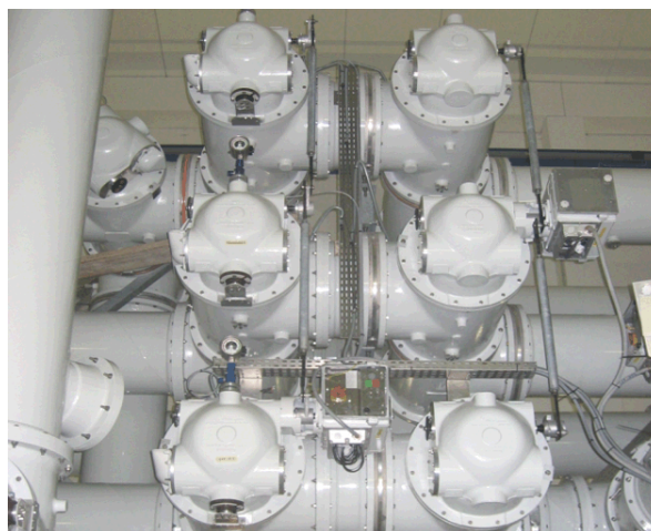
Fig. 1. 400 kV Disconnector in the new Viennese GIS
