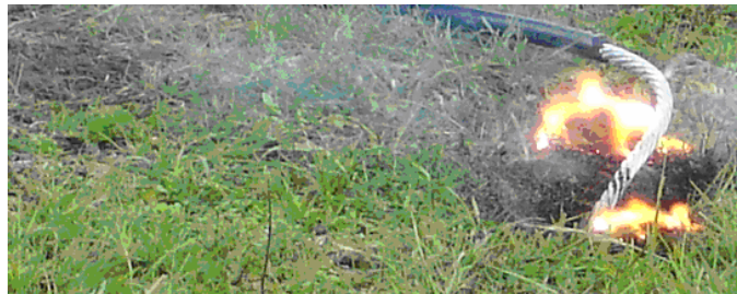
Fig. 14. 13.8 kV conductor in touch with the wet grass.
