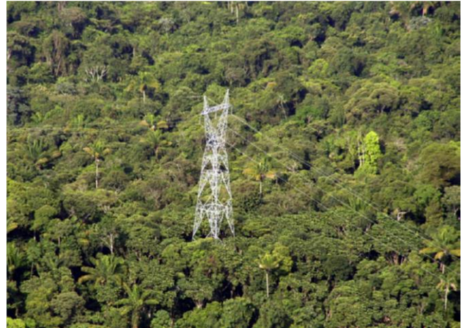
Fig. 1. Transmission tower with 250 meters height into the Amazon forest.
