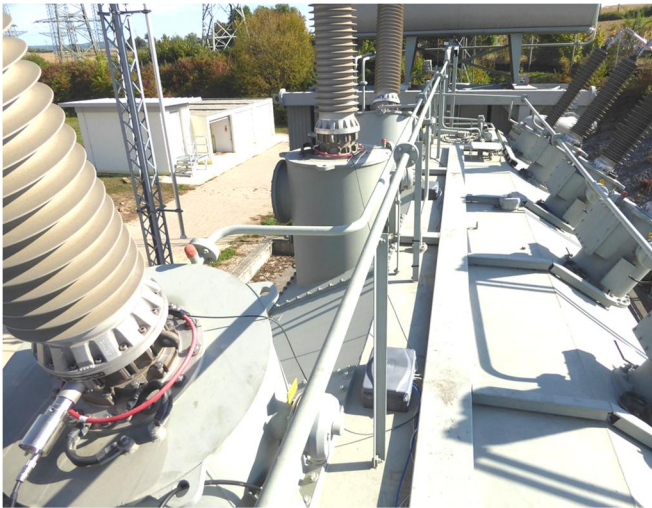
Fig. 3. View of coupling unit connected to the measurement tap of the bushing for the voltage measurement and view of the rogowski-coil used for current measurement
