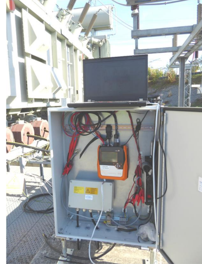
Fig. 4. View of the cubicle installed closed to the transformer, where the PQ device was installed
