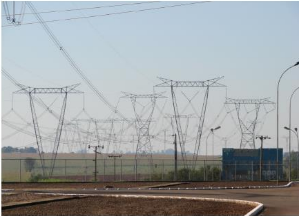
Three AC 765 kV Lines - 6300 MW Foz do Iguaçu Substation
