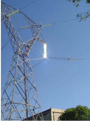
Fig. 2. Former instants of electric arc ignition along the insulator string.
