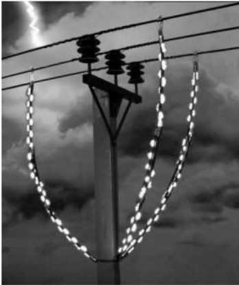
Fig. 15. Protection of 13.8 kV overhead lines against direct lightning strokes by LFA-M arresters [6]
