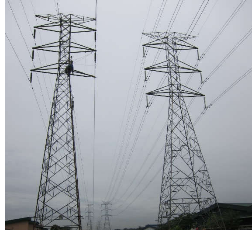
Fig. 3. Installation of FRP crossarms on 132kV (left) and 275kV (right) towers
