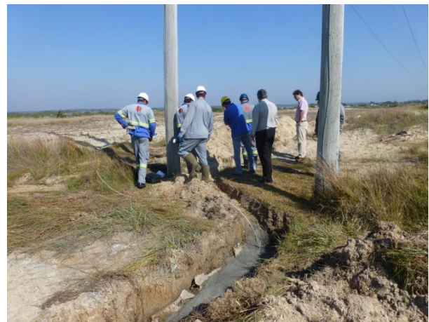
Fig. 12. TL grounding structure encased in concrete.
