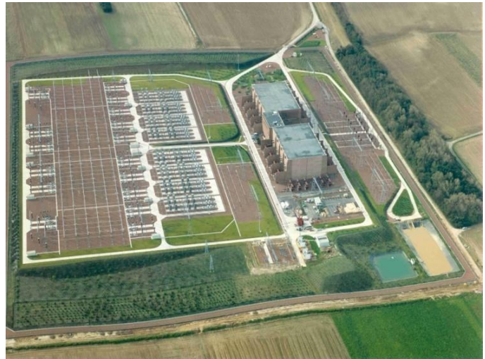
Fig. 1 Aerial view of the IFA2000 substation
