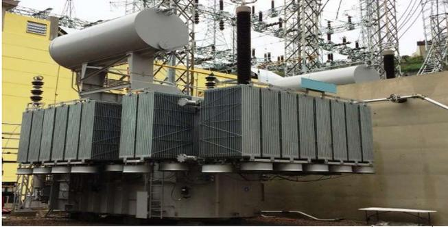
Fig. 1. Single-phase power transformer 200MVA,  $500 / \sqrt{3} / 138/\sqrt{3} / 13.8$  kV installed closed to a GIS substation.
