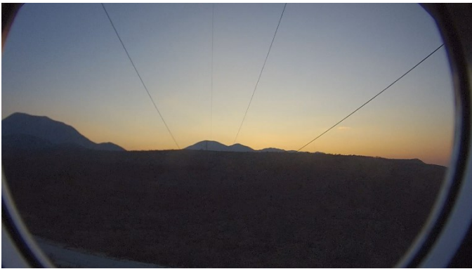
Fig. 13. View from the IP camera installed on tower no. 38.
