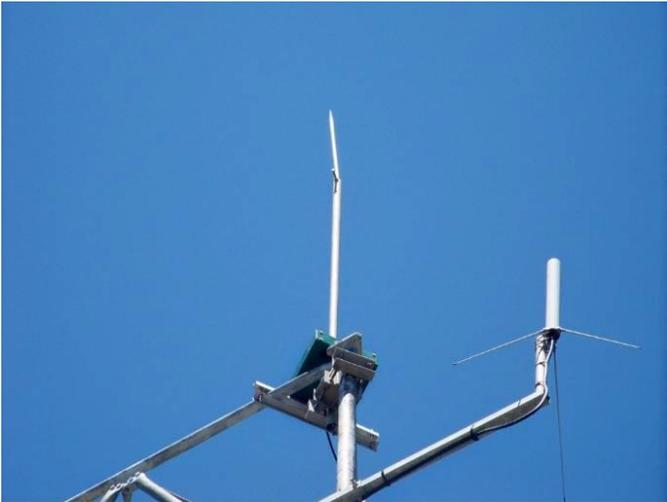
Fig. 1. Current transformer installed at the lightning rod of the telecom base station Miluccia in Corsica (photo taken from [2]).
