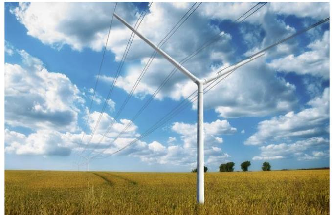
Fig. 1. The concept appearance of the Y-shaped pylon used for 400 kV transmission lines.
