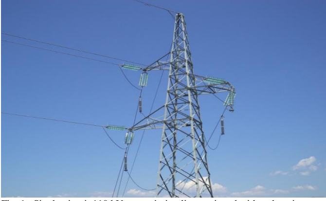
Fig. 1. Single-circuit, 110 kV transmission line equipped with a sky wire
